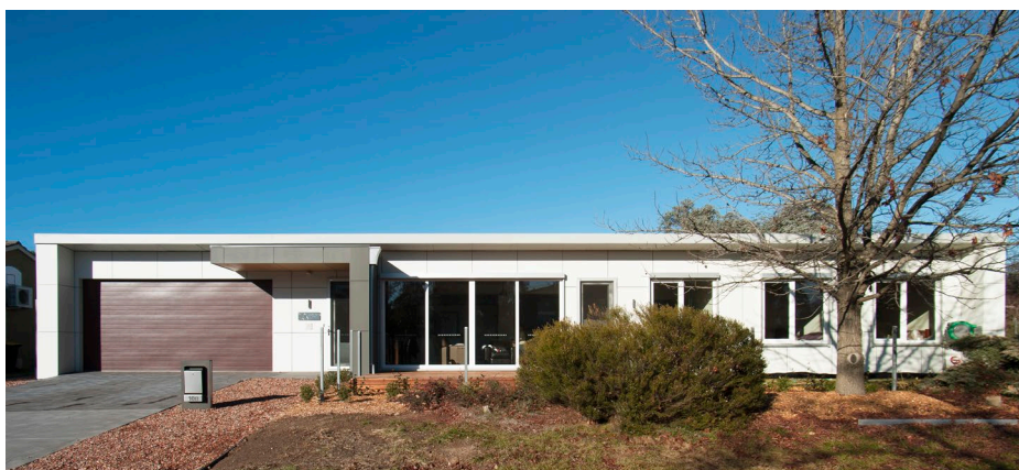
↑ Harley's Passive House, front (north-facing) elevation. Harley built two almost-identical three-bedroom homes on the 1020 m 2 site, each optimised for passive solar gains.
