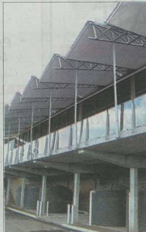
• A rainwater harvesting system has been integrated into the extension where half a dozen tanks underneath the veranda collect rainwater to be used to flush toilets.
