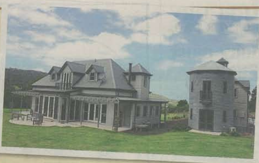
■ Rural house, Foxground (BHI): The house overlooks rural pasture and rainforest escarpment. The architecture is a collection of "farm" buildings in a contemporary and ordered manner. It includes the main house, the silo building used for guests and as a studio, and the barn for guests and a garage. The materials and colours selected reinforce the rural character.
