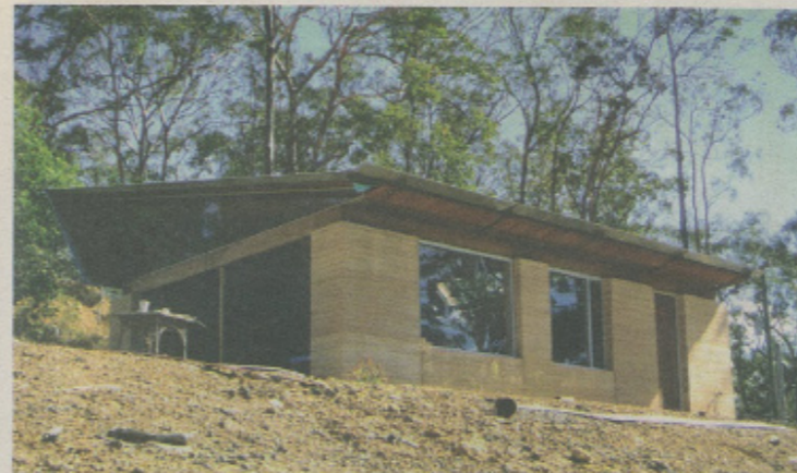
Feat of clay Rammed earth, poured into formwork, gives this house designed by Caroline Pidcock a warmly textured finish. The contemporary style demonstrates why architects are embracing these age-old methods.
