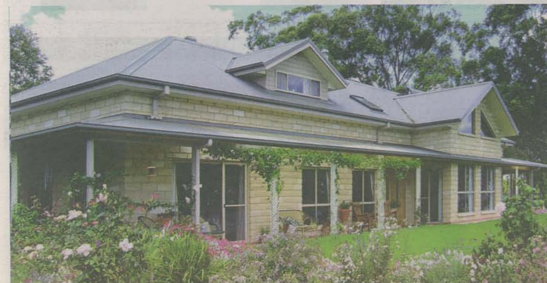
Beauty on a budget At first glance it looks like sandstone, but this house is in fact made of the highly fire-resistant and practical Timbercrete blocks.
