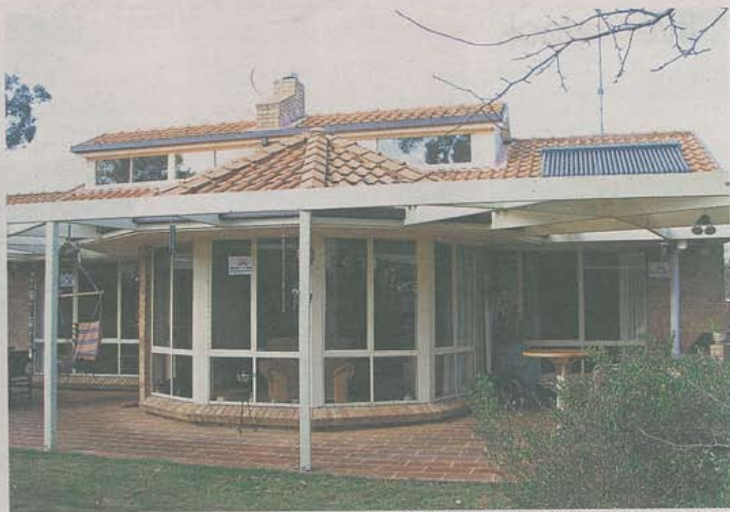
THE LEVER HOME, AN AWARD-WINNING ECO-FRIENDLY HOUSE AT GLENHAVEN, WILL BE OPEN FOR THE SUSTAINABLE HOUSE DAY EVENT.
